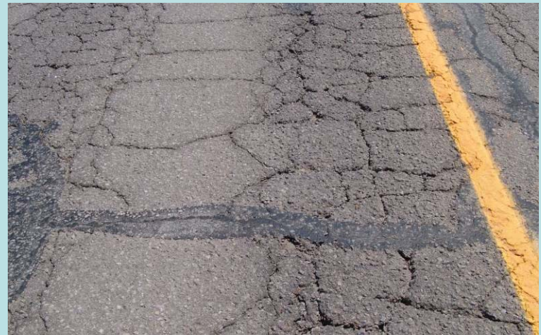
Alligator cracking on SH 90
