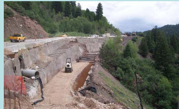
Keystone Hill climbing lane under construction
