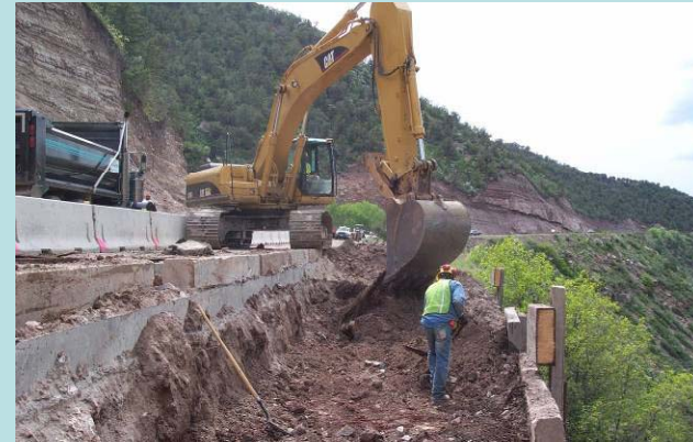
Norwood Hill failed cribwall repair
